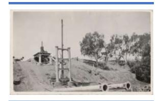
The excavations for the base of  $6'^{11}$  diameter and  $25'^{12}$  into the river bed belled out to  $8'^{13}$  at the bottom. Water pumps were used to keep the water level down during excavation.
