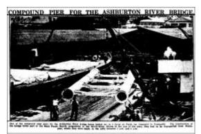
Main Roads ordered four compound steel piers for the bridge made at the Welshpool factory of Forward Down and Co. They were 30 feet long and 15 feet<sup>9</sup> wide weighing about seven tons each. They were carried as deck cargo on the MV *Kangaroo* on four trips by the end of 1930<sup>10</sup>
